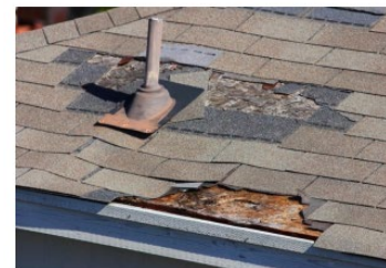
Figure 2. Damaged Shingles and Rotted Roof Deck. (Source: mullinsgc.com)
