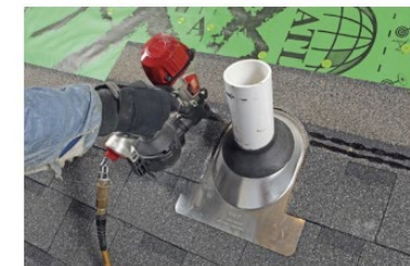
Figure 3. Integrating Roof Penetration Flashing with Shingle. (Source: finehomebuilding.com)
